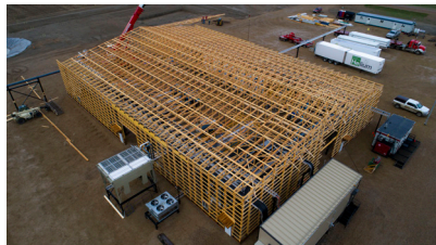
© North American Helium | Battle Creek under construction earlier this year
